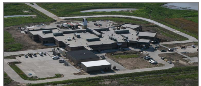
Aerial view of new Community Medical Center
